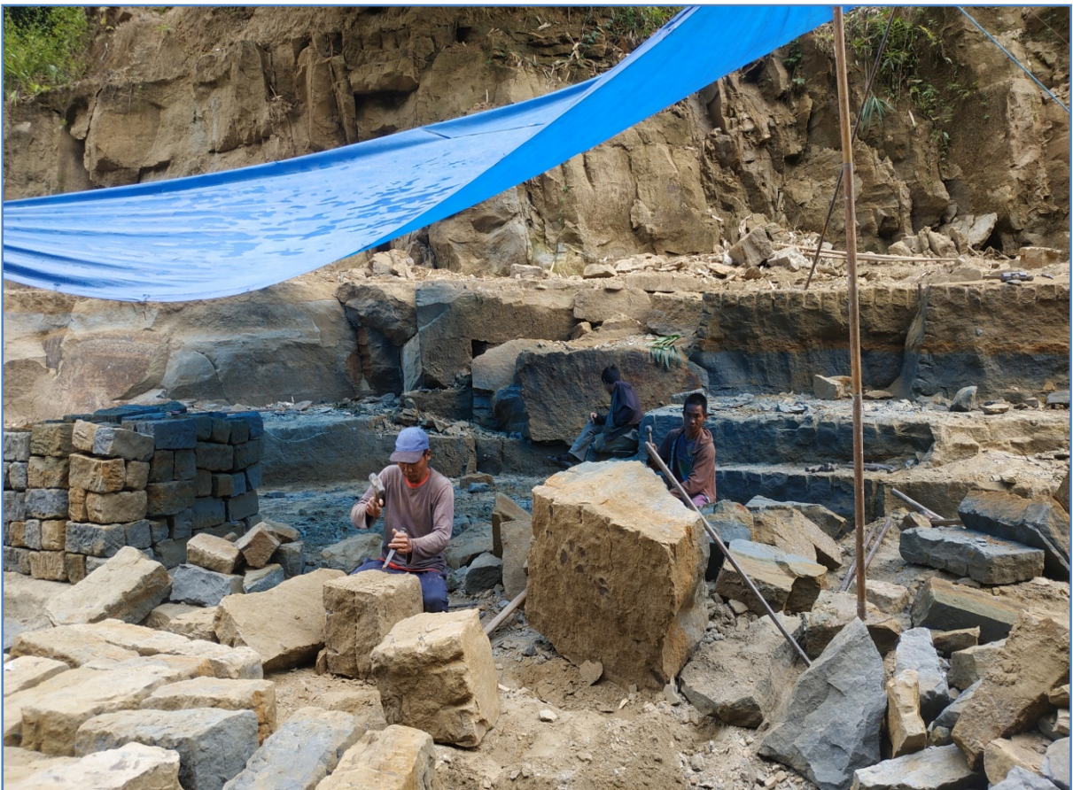
Fig.4: Making Block for Construction at Tuichang River
