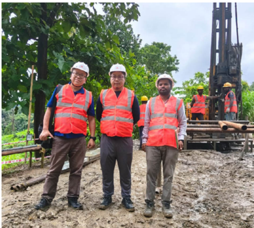
Last borehole MRW-15 (PBH-03). Drilling finished on 31st July 2025f Rotlang West, Lunglei District
