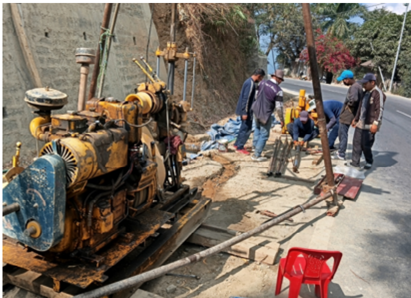
Core Drilling at Hunthar
