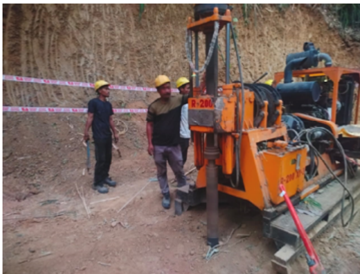
First borehole, MRW-01 (P-05) spudding on 13 th March 2025R at Rotlang West, Lunglei District
