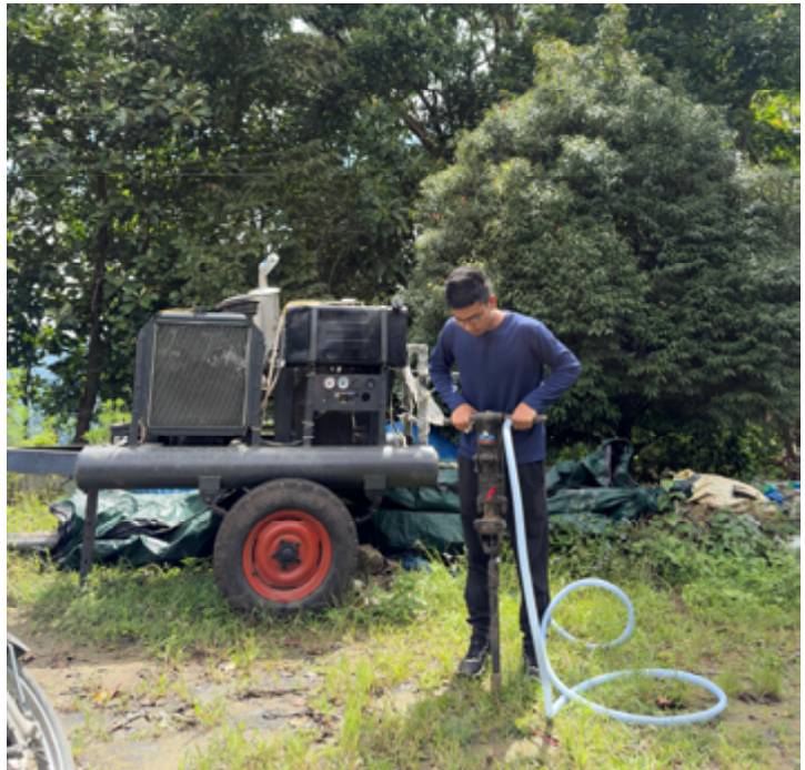
Rock bolting machine with compressor
