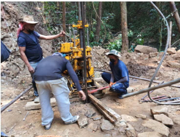
Core Drilling at Vankal
