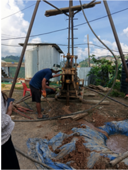
Core Drilling at Lawngtlai
