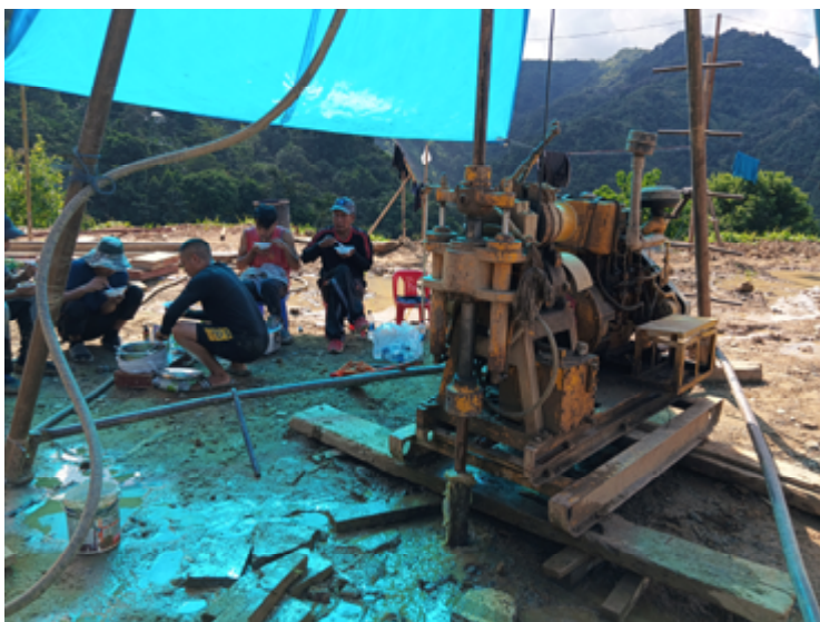
Core Drilling at Bungbanga
